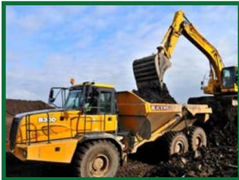
Working for Stewart Milne Homes, Blackwell prepared the site for use as a residential development by uncovering and treating approximately 50,000m<sup>3</sup> of contaminated waste. The development of the land was programmed to commence before remediation operations to treat the contaminated substances were complete. As such, the remedial works were undertaken in four phases.
