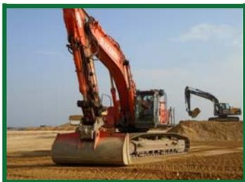
Working for the joint venture, Blackwell carried out specialist earthworks and associated work packages to support the construction of the facility for mooring vessels at Alexandra Dock. Blackwell's scope of work included the removal of redundant site apparatus, bulk earthworks and the creation of a capping layer to produce a strong foundation for the new facility.
